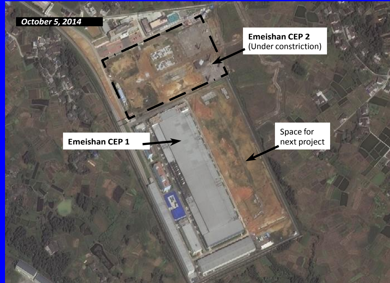
Satellite image from October 5, 2014 (Coordinates: 29°40'38.33" N/103°32'04.65" E). The image shows CEP2 under construction. Source: DigitalGlobe
